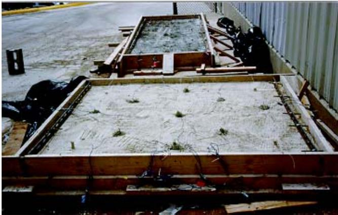
Figure 5-9(b) Thermocouple layout before casting overlay
