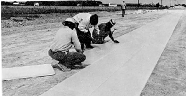
Figure 2.4 Styrofoam insulating layer used on graded subgrade for flexible pavement
