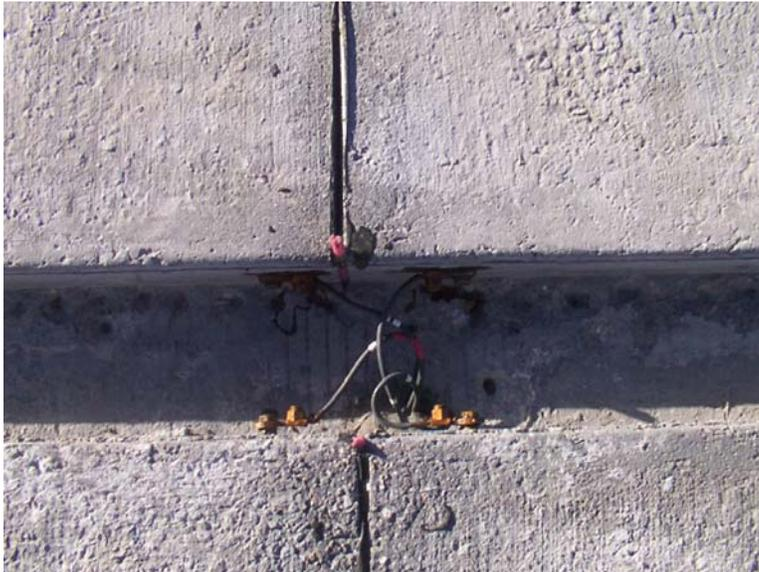
**Figure 6-6 Power Chord and Angle Iron Connection**
