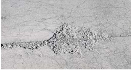
Figure 2.1 D-line cracking spreading from sidewalk joint
