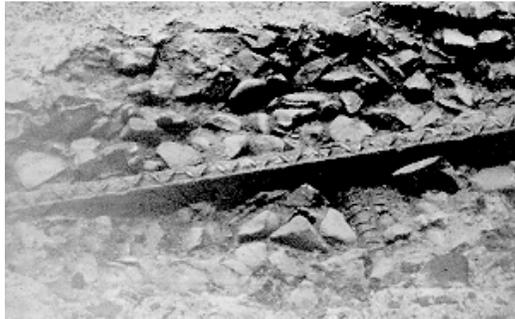
Figure 2.2 Spalling of concrete surface, exposing a reinforcing bar
