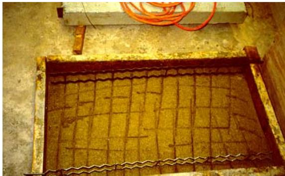
Figure 3-18 Sawdust layer was used as insulation layer
