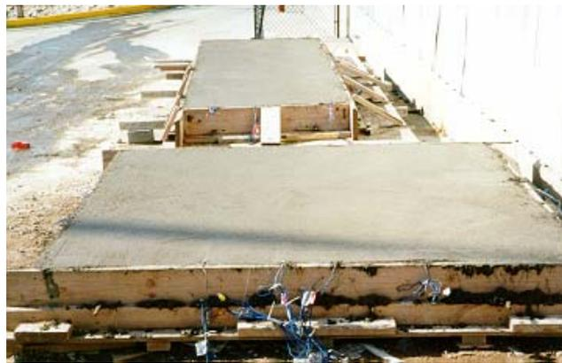
Figure 5-6 Slabs after finishing
