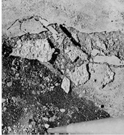
Figure 2.3 Scaling of concrete slab surface
