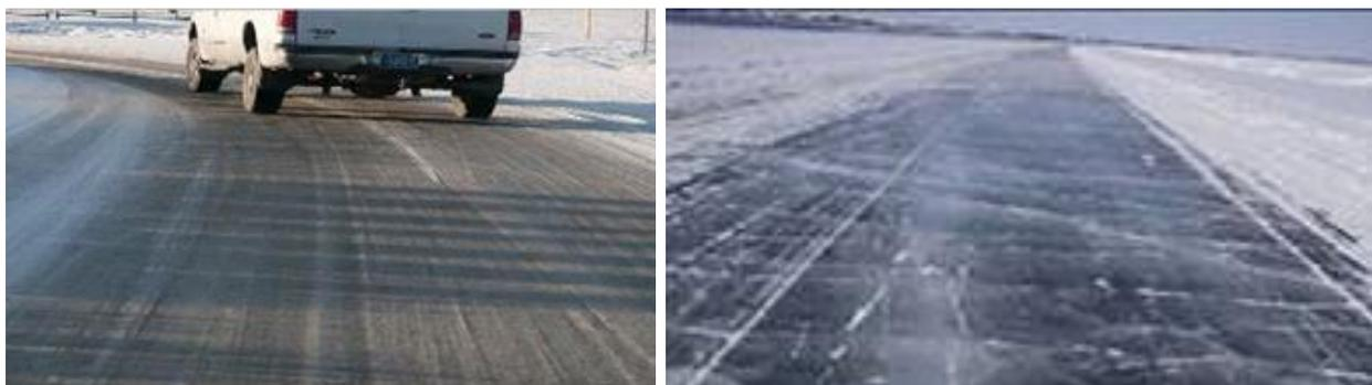
**Figure 7 Examples of “black ice” road conditions (Veneziano et al., 2014; photos courtesy of WTI and MDT).**
