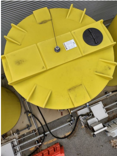
Figure 6. Storage Tank Radar Level (Source: Marc Valenti)
