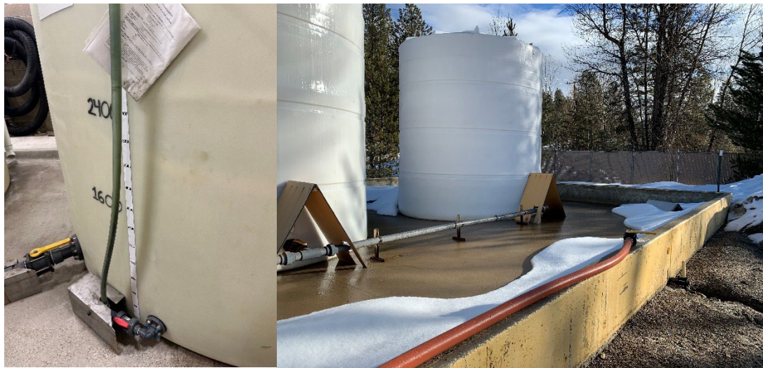
Figure 4. Storage Tank Plumbing Coverings (Source: City of Farmington Hills, Mi – Left, Idaho Transportation Department – Right)
