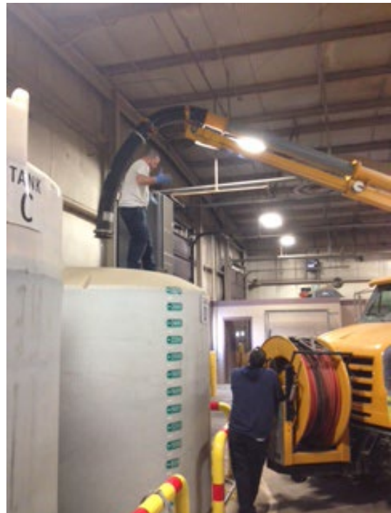
Figure 19. Poly Storage Tank Cleaning (Source: City of Farmington Hills, MI)
