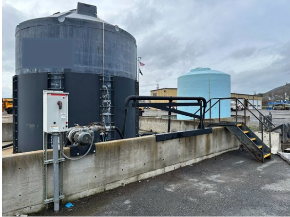
Figure 24. Oregon Department of Transportation Tank Farm, The Portland Metro Area maintenance yard pilot tested the use of salt brine in the 2023-2024 winter season.
