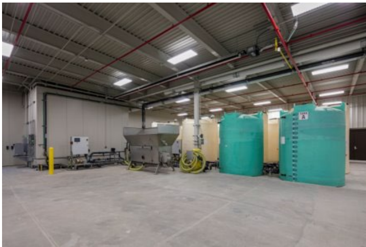
Figure 26. City of Farmington Hills, MI Indoor Liquids Facility (Source: City of Farmington Hills, MI) has an indoor truck fill with two fill points (top left), storage tanks and brine maker (bottom left), and storage tank plumbing (right). City of Farmington Hills, MI uses MP pumps on “stacked” three product fill point systems, as well as their brine making system.
