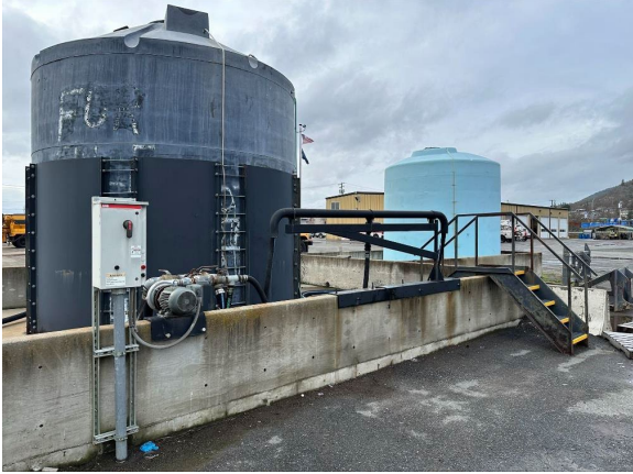
Figure 10. Concrete Containment Wall (Source: Oregon Department of Transportation)
