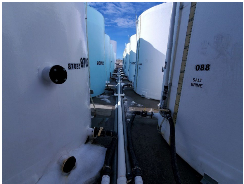
Figure 3. Storage Tank Plumbing with Valving for Shut-Off (Source: Nebraska Department of Transportation)
