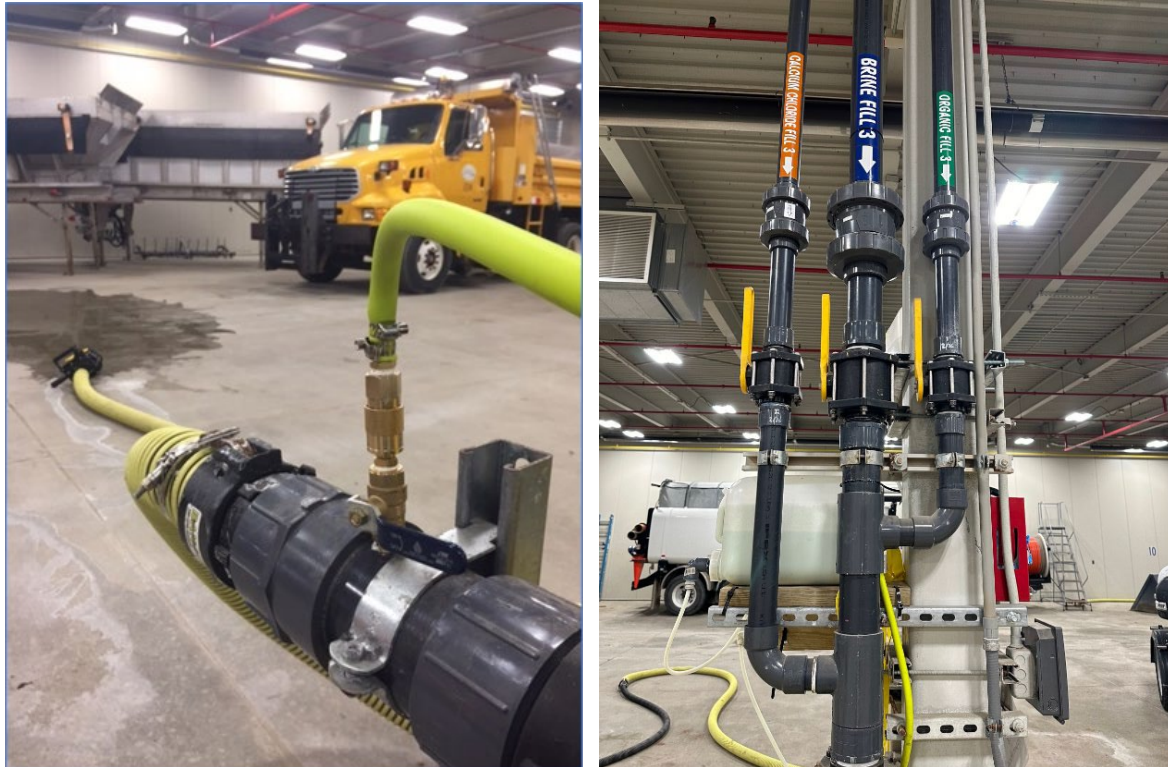
Figure 20. City of Farmington Hills—Air Purge for Fill Hoses (Left) and One-Way High Flow Valves (Right); (Source: City of Farmington Hills, MI)
