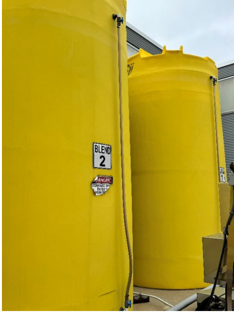
Figure 5. Storage Tank Sight Tube (Source: Marc Valenti)
