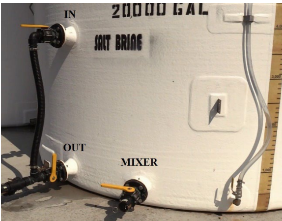
Figure 25. Kansas DOT Tank Farm Utilizing Fiberglass Tanks (above). Kansas DOT will manually blend as needed and is uses a truck fill with a single flow rate. The fiberglass tanks have a port at the center of the base of the tank that is used for mixing or recirculation of materials (bottom left). The port has three peri jets inside the bottom of the tank to help circulate material (bottom right)
