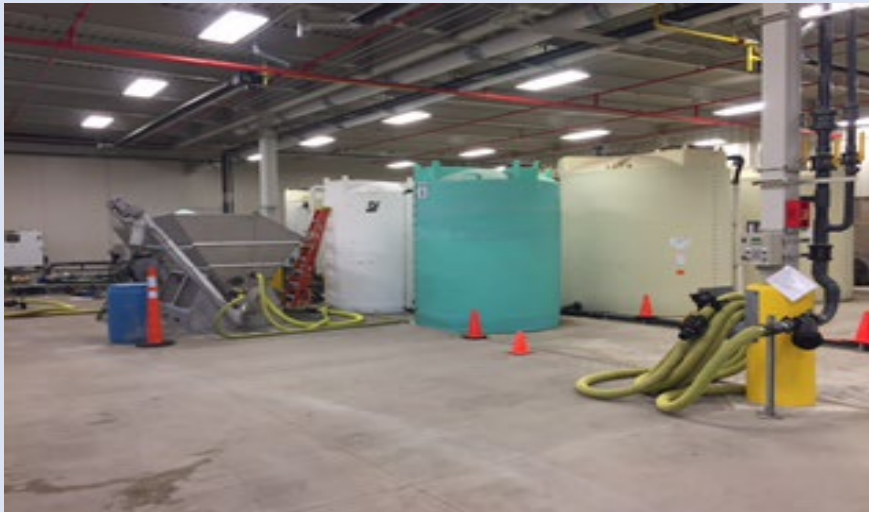
Figure 7. City of Farmington Hills, MI Liquids Manufacturing Room—Storage Tanks (Source: City of Farmington Hills, MI)
