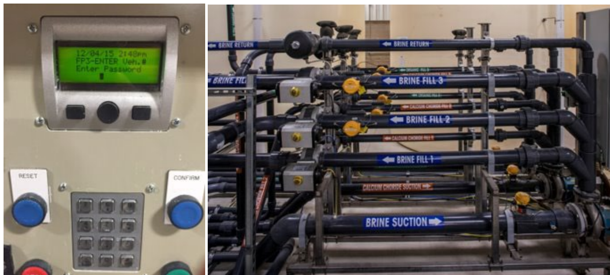
Figure 27. City of Farmington Hills Login Interface That Allows Data Recording for Vehicle, User, and Product or Blend (Left) and Automated Blending of Three Products with Anti-Foaming Agent (Right; Source: City of Farmington Hills, MI)
