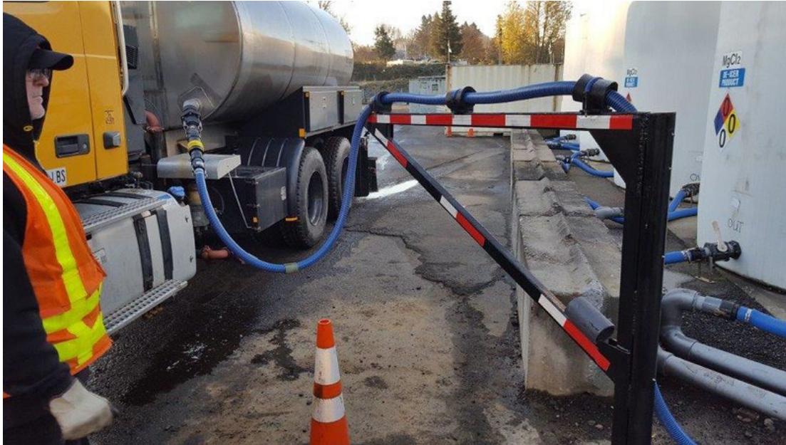
Figure 14. Fill Point Hose Attached to Swing Gate (Source: Oregon Department of Transportation)
