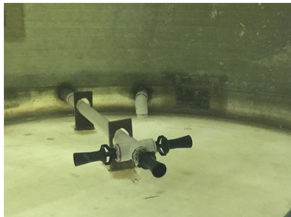
Figure 25. Kansas DOT Tank Farm Utilizing Fiberglass Tanks (above). Kansas DOT will manually blend as needed and is uses a truck fill with a single flow rate. The fiberglass tanks have a port at the center of the base of the tank that is used for mixing or recirculation of materials (bottom left). The port has three peri jets inside the bottom of the tank to help circulate material (bottom right)
