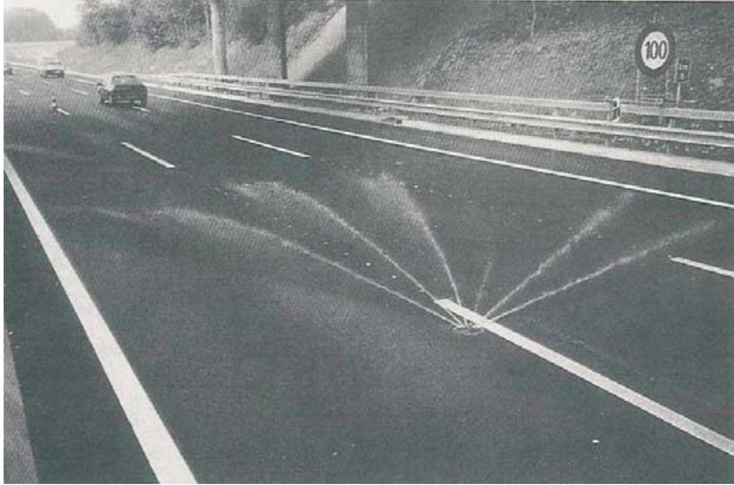
Figure 7: Spray head in action from a FAST system (Zhang et al. 2007)
