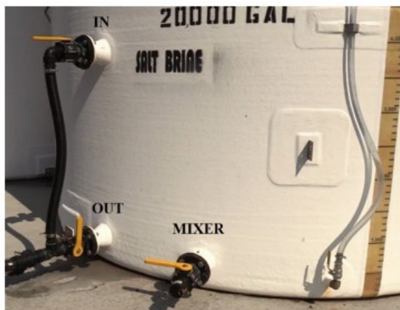
Figure 25: Tank Mixing Port and Peri Jets Inside the Bottom of the Tank
