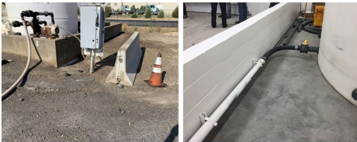
Figure 21: Liquid Deicer Storage and Pump System Secondary Containment Concrete Wall
