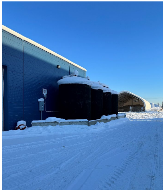
Figure 13. Liquid Deicer Storage Tanks
