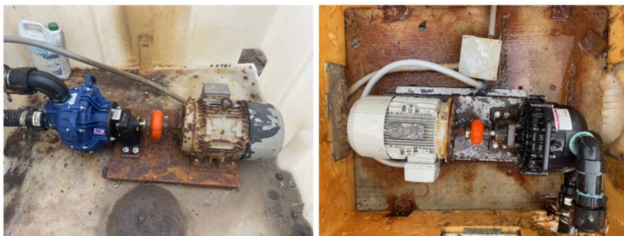
Figure 34: Pumps with Lovejoy Connection to the Motor (John Blue Pump - Left, Banjo Pump - Right)
