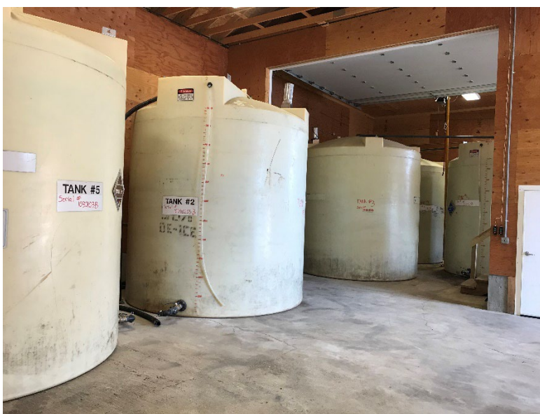
Figure 28: Liquid Deicer Storage Tanks
