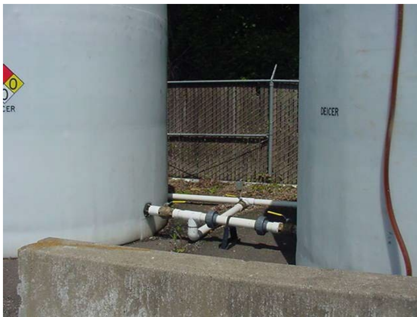
Figure 32: PVC Plumbing of Liquid Deicer Storage Tanks.
