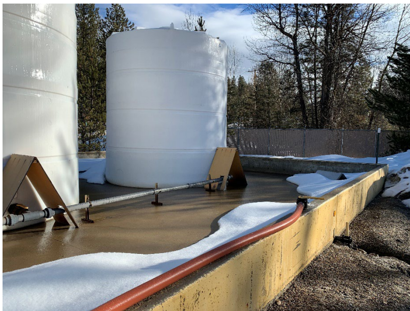
Figure 22. Coverings for System Plumbing
