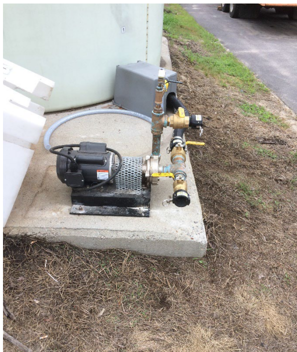
Figure 27: Pump/Motor Set Up on Metal Plate
