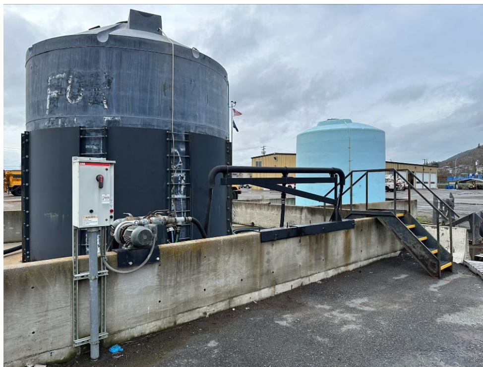
Figure 33. Storage Tank with Secondary Containment Retention Wall
