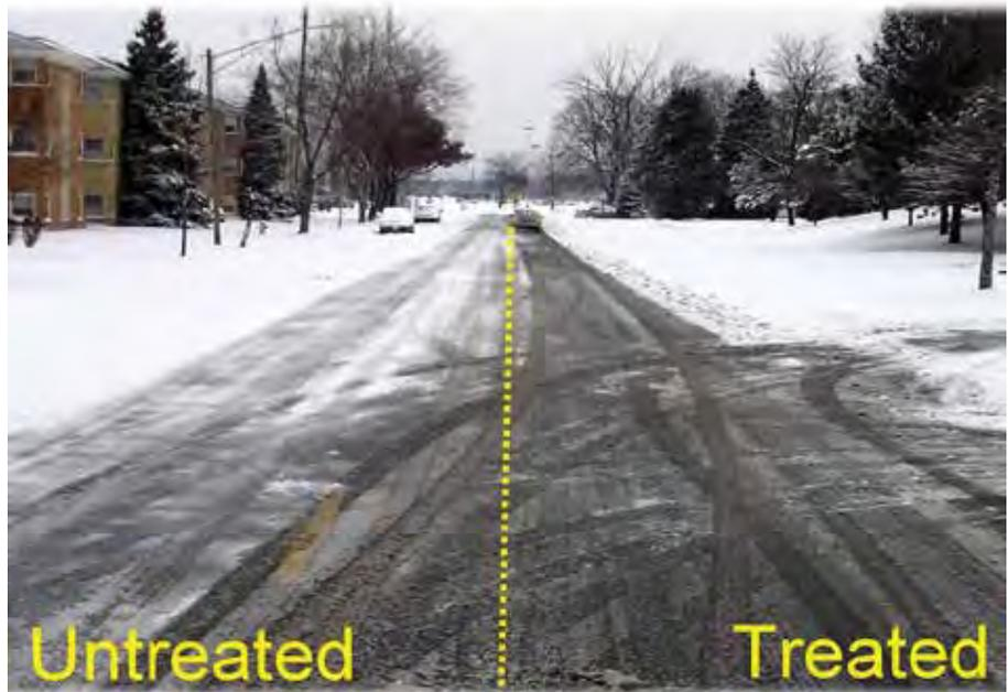
**Photo#3: Anti-icing can reduce salt usage by up to 75 percent if conditions are right. The manual includes a flowchart to help determine whether anti-icing is likely to be effective.**
